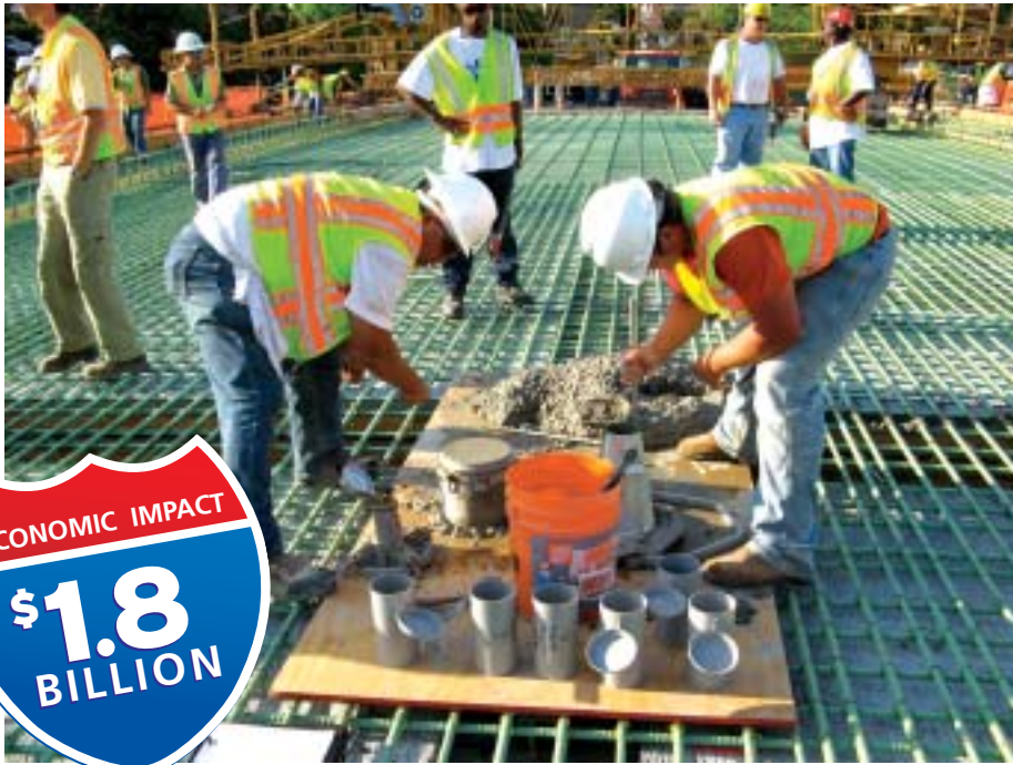
Quality Control inspectors test a batch of concrete to make sure it meets specifications.
